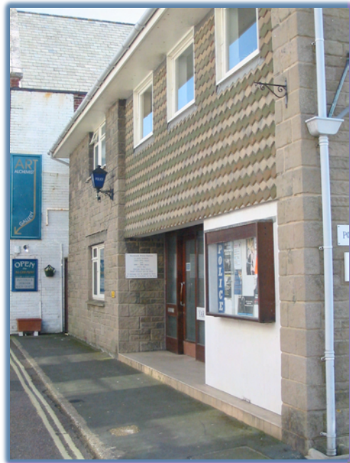
Yarmouth Police Station © BCE
